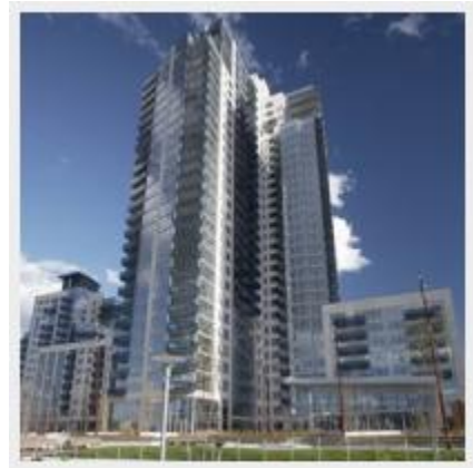
This view of The Edge is from the waterfront esplanade. Photo by Jesper Norgaard
